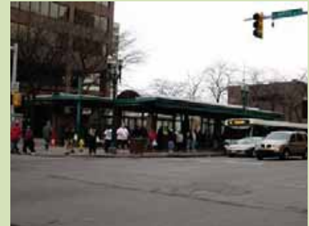
Downtown Bus Station
