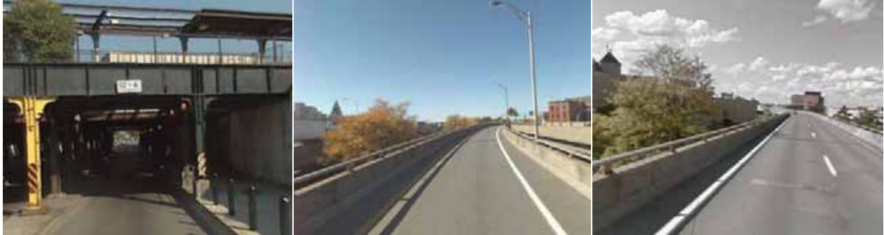
Vertical Clearance Posting and Narrow Shoulder examples
