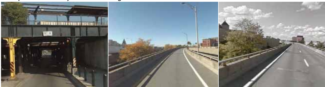
Vertical Clearance Posting and Narrow Shoulder examples
