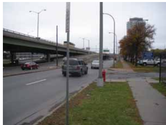
Viaduct looking south
