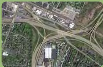
I-490/I-590 interchange, Rochester, NY
