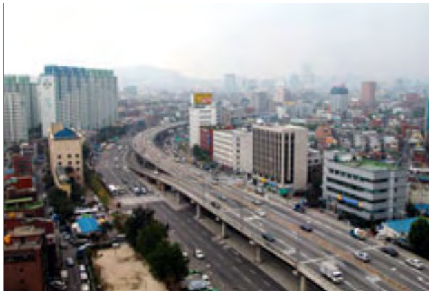
Before: Cheonggyecheon Freeway
