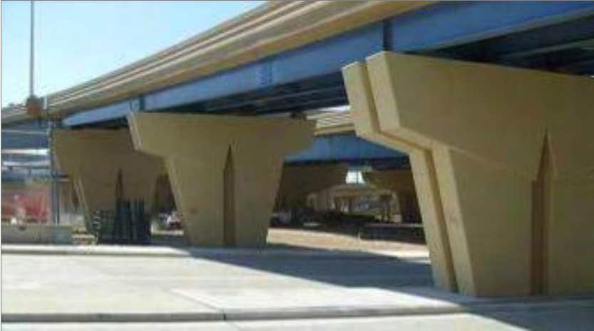
Highway structures emphasized clean lines and light/bright colors
