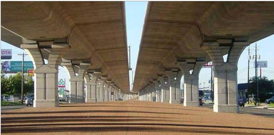
View from under the viaduct. Source: www.texasfreeway.com
