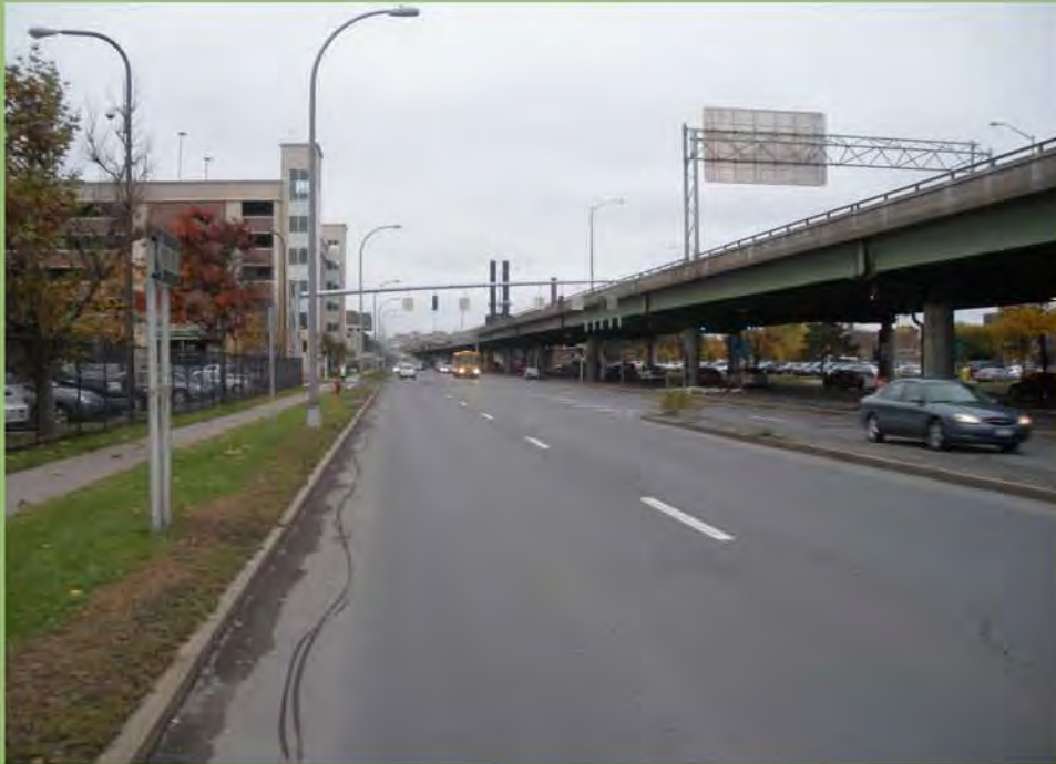
I-81 existing conditions, view south
