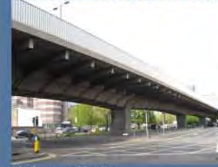
Modern steel bridge Hammersmith flyover, West London
