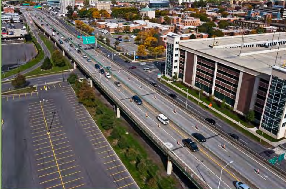
I-81 existing conditions, view north
