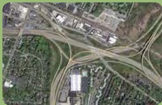
I-490/I-590 interchange, Rochester, NY
