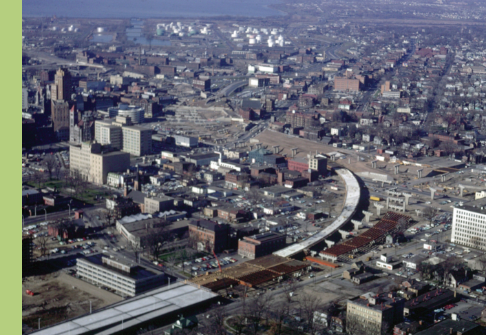
Construction of I-81 through the City of Syracuse
